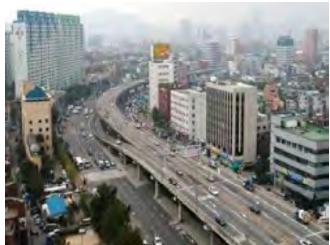
Before: A concrete highway covered the Cheonggyecheon River. It added more traffic congestion.
